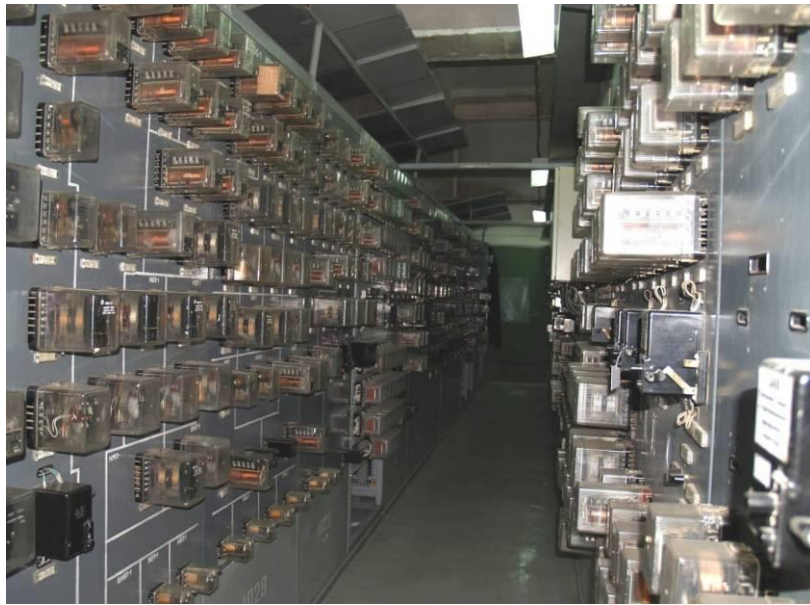
NPP I&C before upgrade by Radiy
