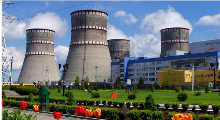
Rivne Nuclear Power Plant, Ukraine
